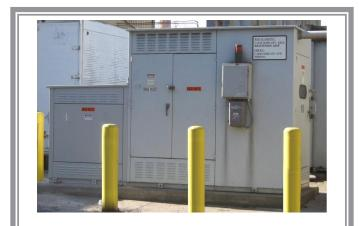
Conversion of 4.16 kV, 1200 kvar Capacitor Bank to 1900 kvar, 4<sup>th</sup> Harmonic Filter Bank
