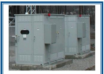
12.47 kV, 4<sup>th</sup> Harmonic Filter Banks – Each with Two 1200 kvar Steps
