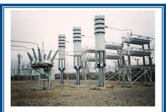
138 kV, 62 Mvar, 5<sup>th</sup> Harmonic, Open Air Filter Bank
